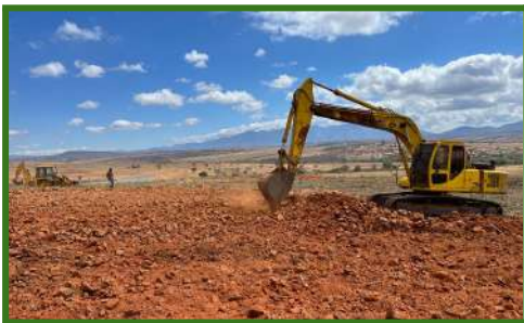
Farm leveling and stones removal
