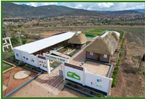
Children's Farm facility construction complete.
